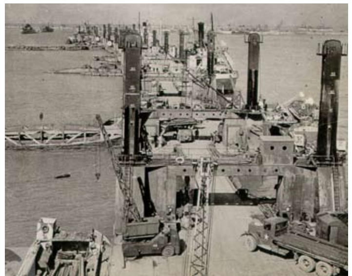
Wharf formed of seven pierheads in a line', showing a view along the line of the Mulberry Harbour Spud pierheads at Arromanches, Gold Beach
