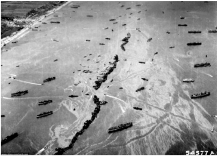
Mulberry Harbour, Omaha Beach. Row of Blockships in place, 15 June, 1964.
