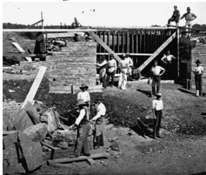
Eastern Battery, Fort Clarence under construction on promontory in Dartmouth overlooking George's Island, 1749
