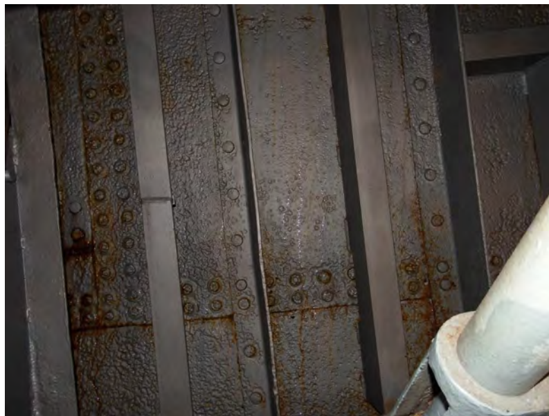
New sister frames inserted between originals to port and starboard.
